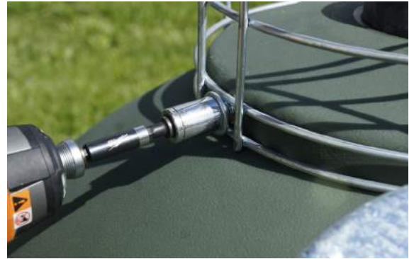
Step 6: Bolt cage to unit.
