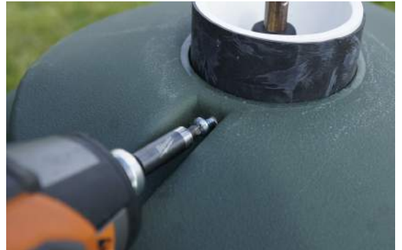
Step 4: Place PVC in hole and attach. (1) Set Screw
