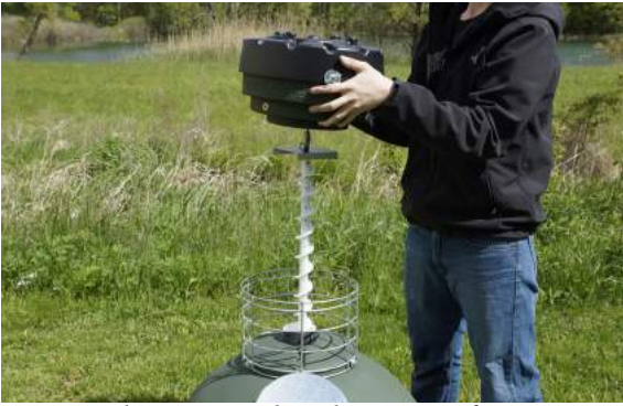
Step 9: Place powerhead on top of cage.
