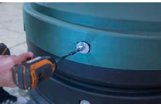
Step 7: Attach dome to extension ring.
